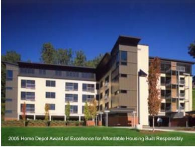
LEEDS certified: high efficiency building envelope; locally cut and milled flooring; state-of-the-art storm water runoff treatment system; advanced heating and cooling systems; direct line of sight to daylight for more than 90% of occupied space.
